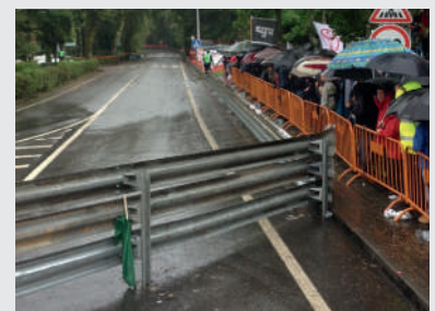
Spectators positioning too close to guardrail
