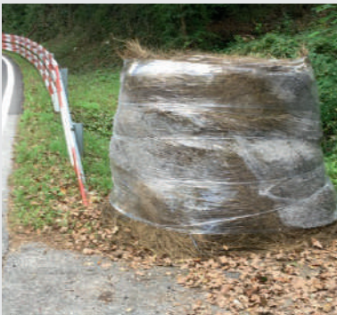
Guardrail nose not protected
