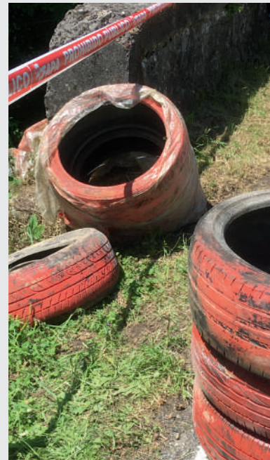
Poorly positioned and constructed tyre stack
